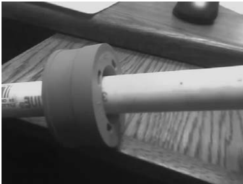
Figure 6. Laundry adapter fitting placed over standpipe.
